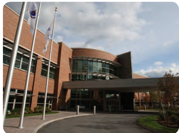
Photo Courtesy of MassDevelopment Finance Agency
