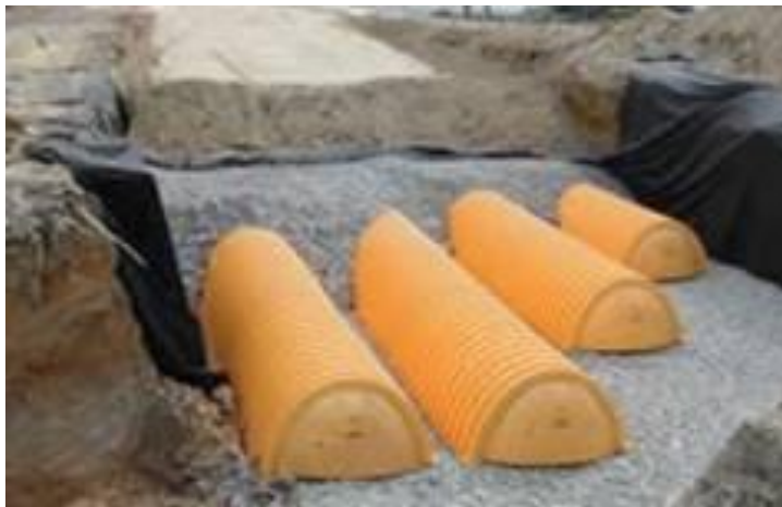
Devens Common underground infiltration systems
