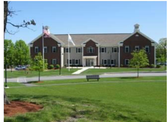
Devens Common cisterns collecting roof runoff
