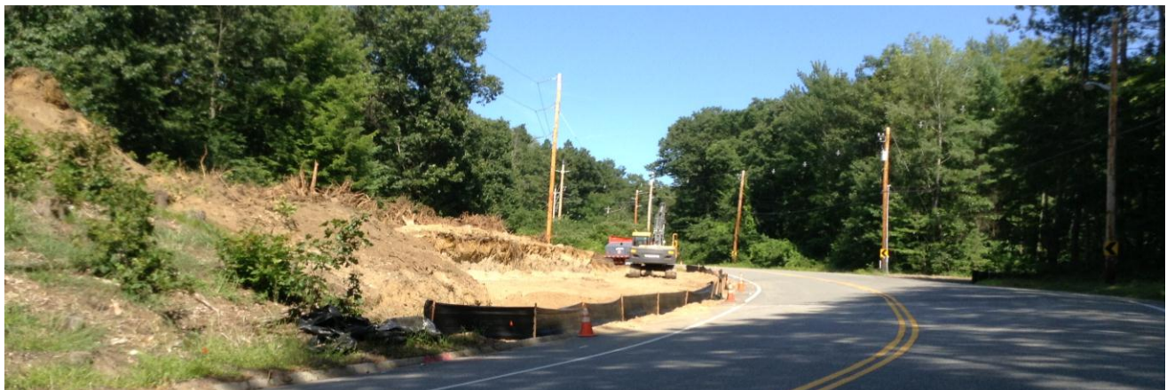
Sight line improvements along Hospital Road – trees removed and slope being cut back to provide safer view for both vehicles travelling down Hospital Road as well as those entering and exiting the new canoe launch parking area – August 2013.
