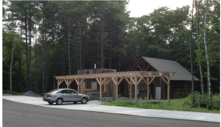
USFWS visitor contact station and parking. Pervious concrete parking area leading to composting toilets and the education pavilion.
