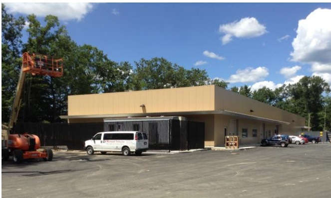
Mill building #1 to the rear of sound stages.
