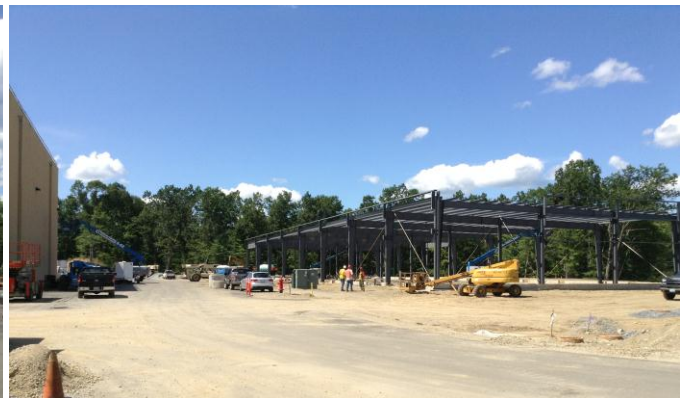
Structural steel erected for mill building #2
