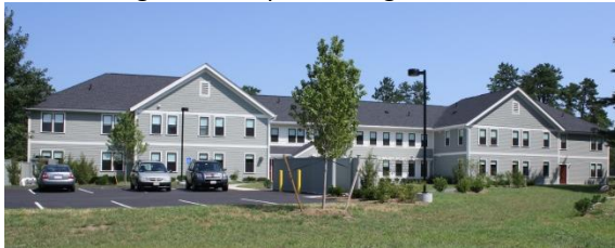
Transitions women's shelter – a 13-unit infill redevelopment for homeless women with children centrally located within a former military residential area that was redeveloped and reused for civilian residents.
