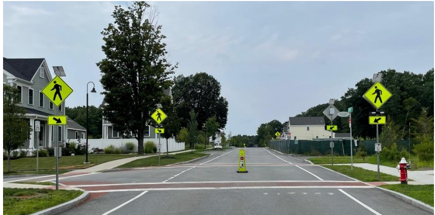
View of Grant Road and the new crosswalk signage and signals at Chance Street intersection. Multi family apartment site surrounded by green construction fencing to the right – August 2023
