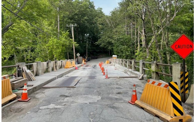
Lovell Road bridge repairs - August 2023
