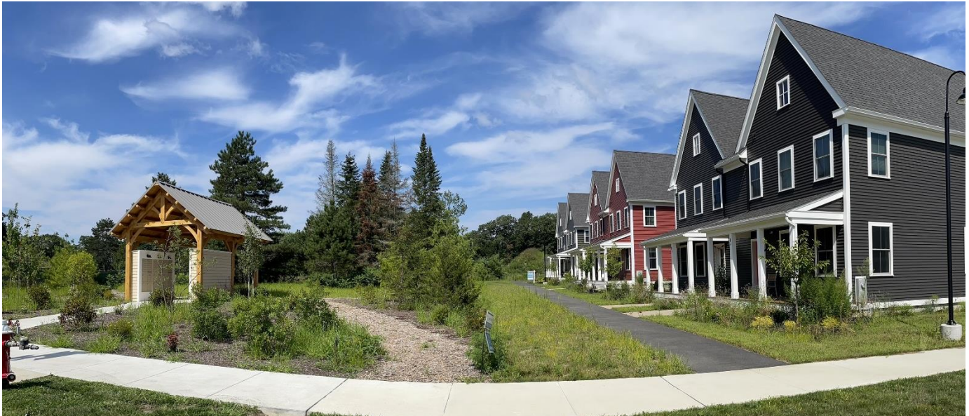
To the right: New Duplexes off of Powell Street fronting on Central Park. To the left: New central mailbox pavilion for the entire Grant Road neighborhood accessible right off of Grant Road - July 2023
