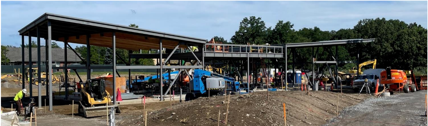
65 Jackson Road – Amenity building structural steel – August 2023
