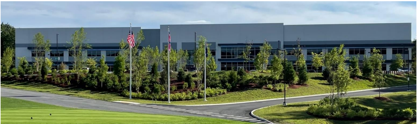
Finished building at 16 Bulge Road– July 2023.
