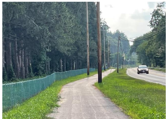
New multi-use path along West Main Street - August 2023
