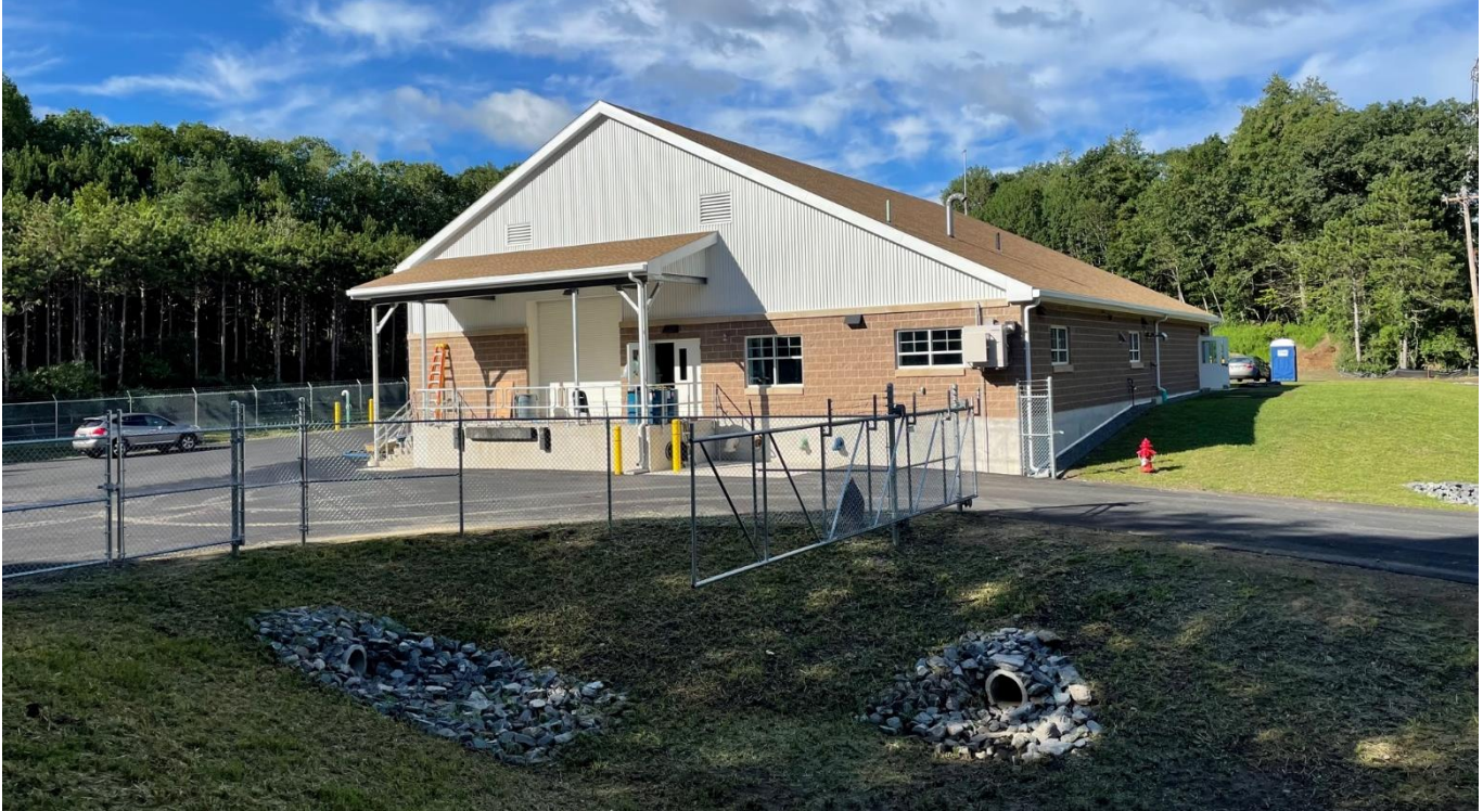
New Patton Well Water Treatment Facility off Patton Road – August 2023
