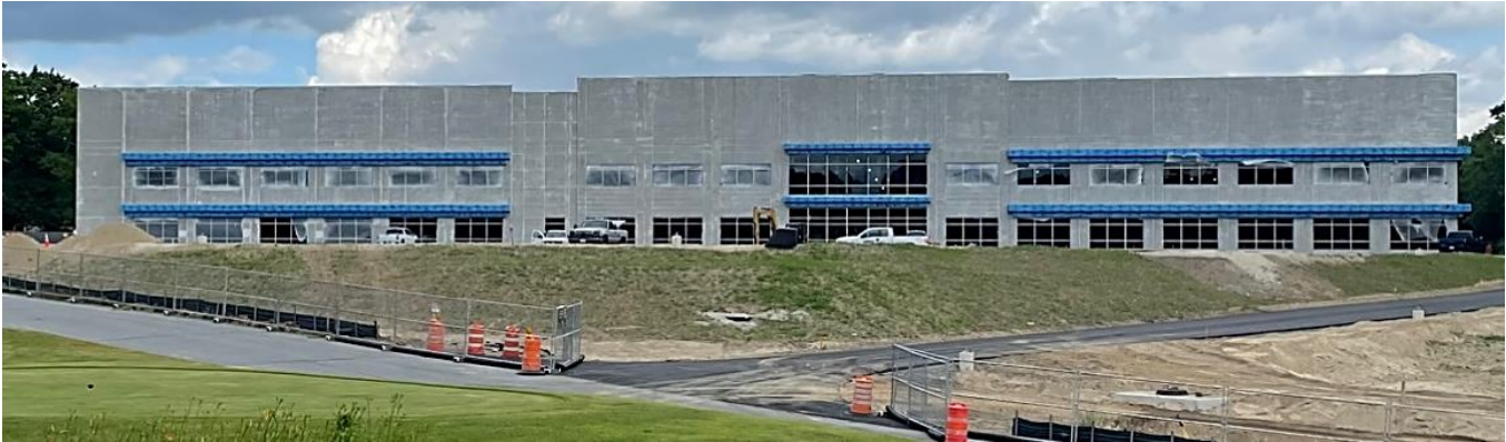
New building at 16 Bulge Road under construction – June 2022.
