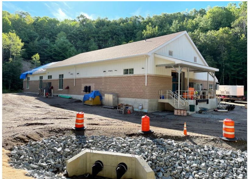
New Shabokin Water Treatment Facility off Sheridan Road: August 2023
