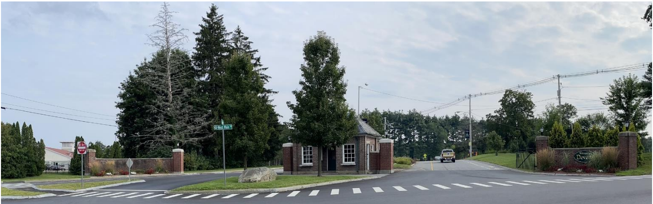
New Landscape islands, bike lanes and pedestrian crossing at the newly restored historic Verbeck Gate – August 2023
