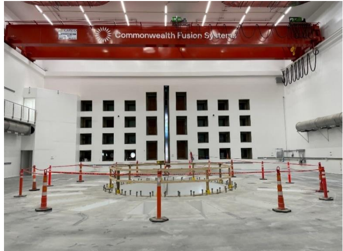
Tokamak Hall nearing completion – August 2023
