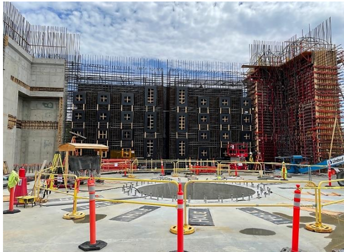
Interior of SPARC – (“Tokamak Hall”) under construction – June 2022
