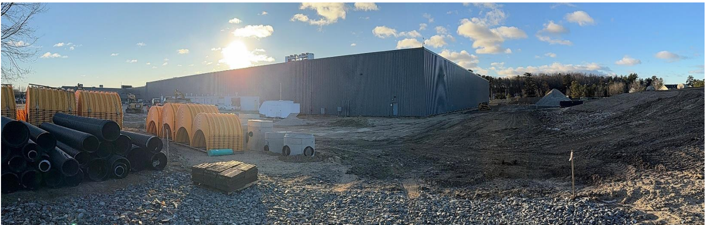
SMC's proposed building expansion underway at 18 Independence Drive. The yellow structures in the foreground are the underground infiltration chambers that will store drainage under the parking lot. – December 2025
