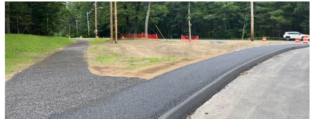
Porous sidewalk and trail connection where old road used to be. June 2024
