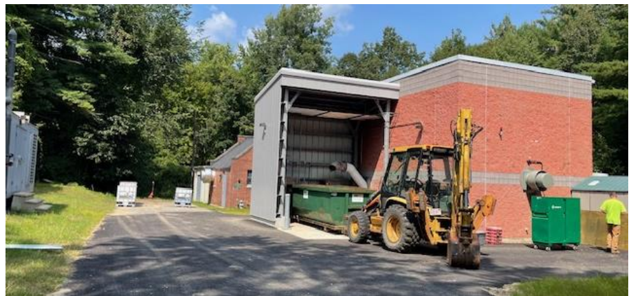
Screenings building addition – MacPherson Road – May 2024
