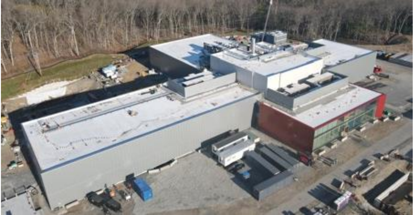
Aerial View of CFS-2 SPARC building– June 2023. Photo courtesy of Commonwealth Fusion Systems.
