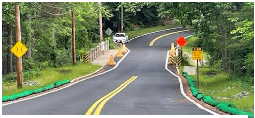
Lovell Road Bridge – June 2024
