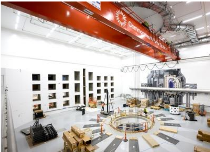
Interior of SPARC – (“Tokomak Hall”) under construction – June 2024
