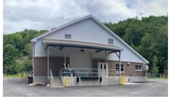
New Shabokin Water Treatment Facility off of Sheridan Road - June 2024
