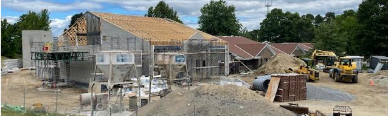
New Public Safety Building under construction – June 2024.
