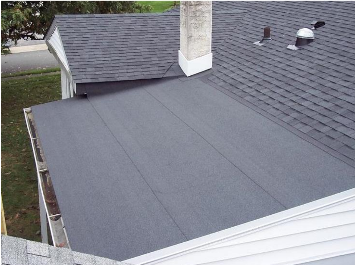
Photo: example of rolled asphalt roofing on a low-pitch roof vs traditional asphalt shingles
