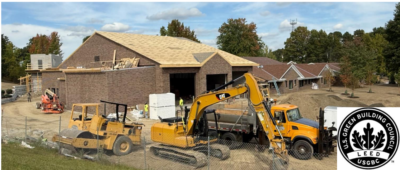
Apparatus Bay at new Public Safety Building – September 2024
