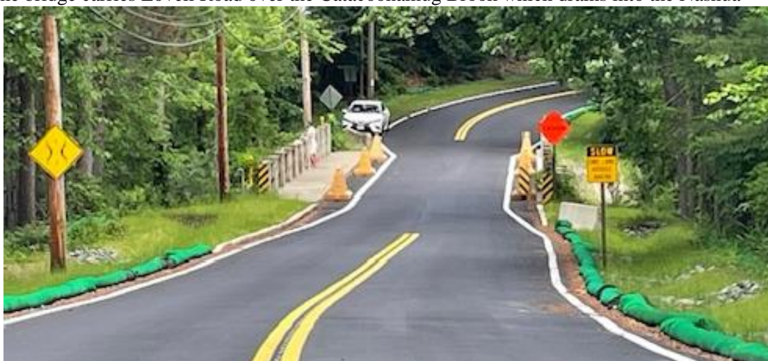
Lovell Road Bridge – June 2024
