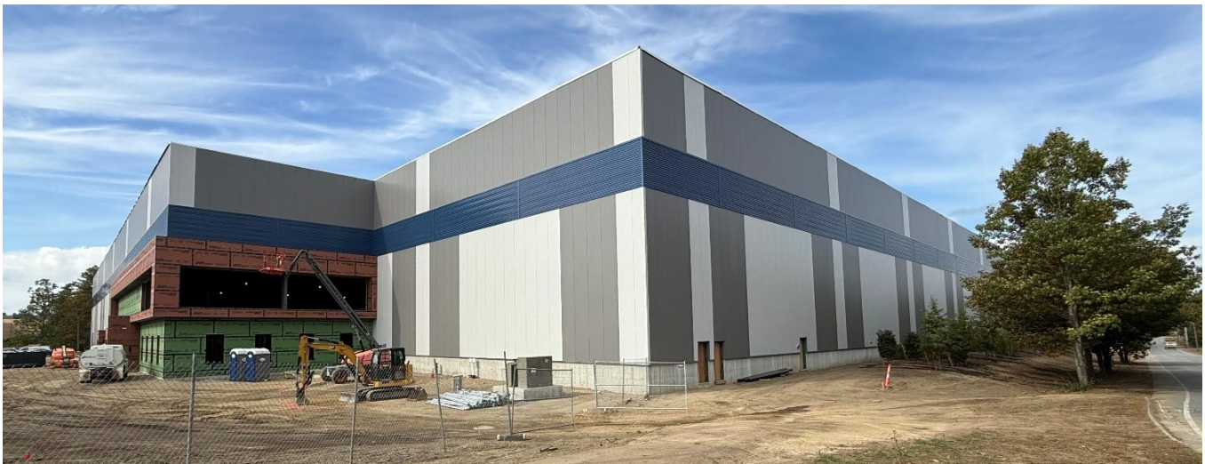
11 Grant Road under construction – September 2024
