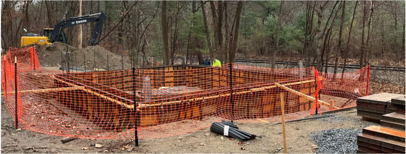
Havard Water Line Booster Pump Station foundation work – November 2024
