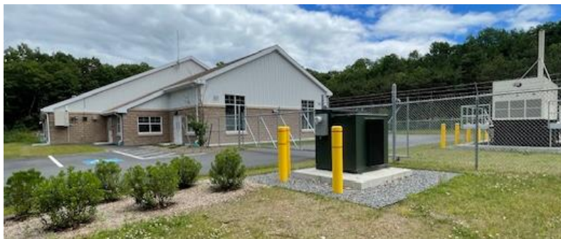
New Patton Water Treatment Facility off of Patton Road
