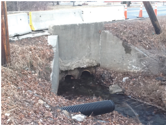
Antietam Culvert before (twin 24" pipes)- March 2012
