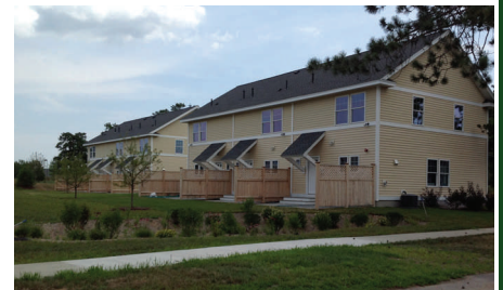
Rear of the first six multi-family sustainable housing units.
