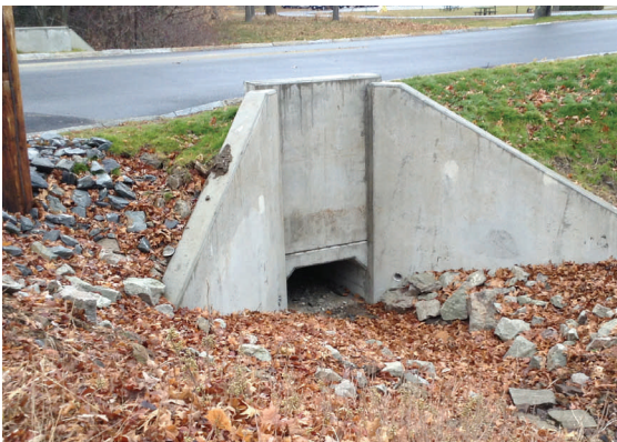
Antietam Culvert after (36" open bottom box culvert, new headwalls)- Nov. 2012
