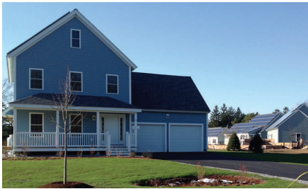
New home on Adams Circle. In the foreground. Rear of new homes along Cavite in the background—adorned with solar panels.
