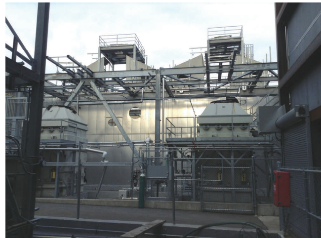
After: all noise generating equipment & process piping removed (Nov. 2012)
