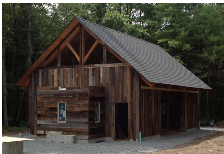
Reclaimed barn siding gives a "rustic" but sustainable finish to the new USFWS Visitors Center.
