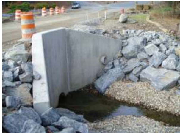
New culvert headwall at Cold Spring Brook
