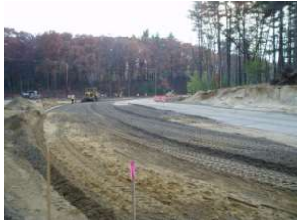
Rough grading of new road alignment
