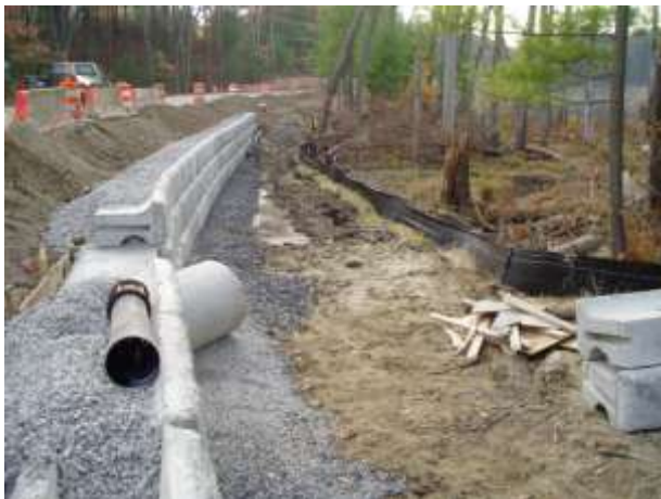
Retaining wall adjacent to disturbed wetland area
