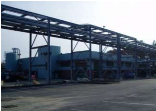
CUB Building and Utility Pipe Rack – October 2008
