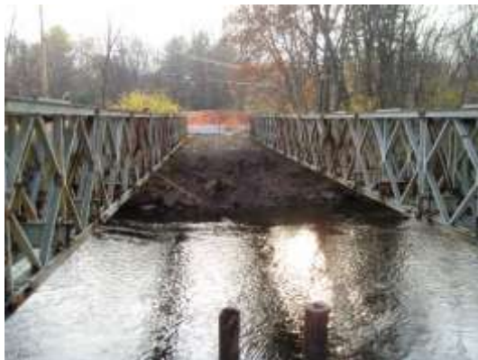
Bailey Bridge with decking and cross beams removed
