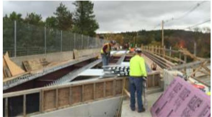
*Jackson Road Bridge over Route 2 – looking north – Northbound lane of bridge decking being installed – October 2016*
